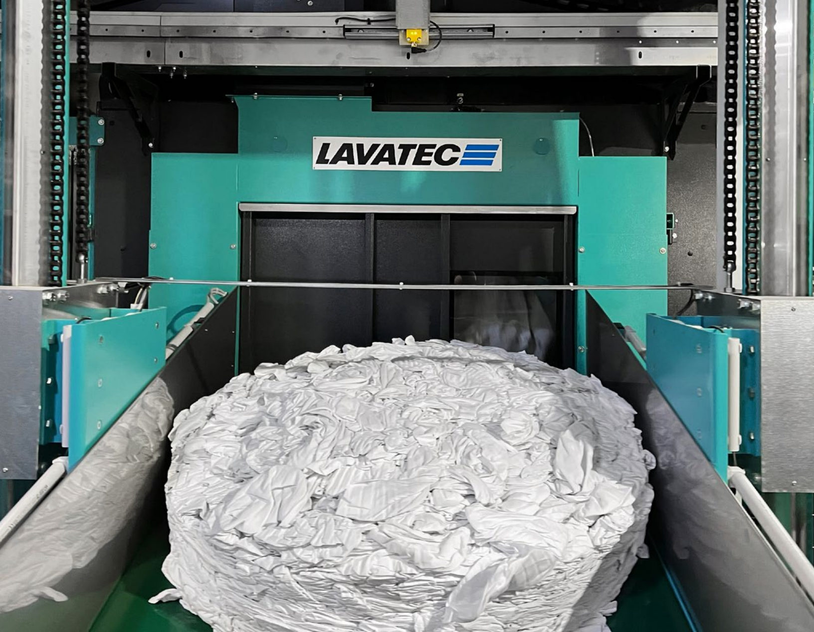
A laundry cake travels from the tunnel washer to its next destination, one of the six new TT-745 gas dryers installed last month.
